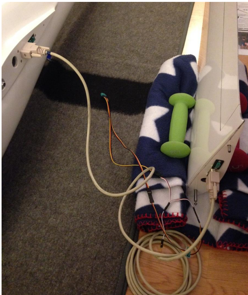
Figure 56. Close up of extension cables.
