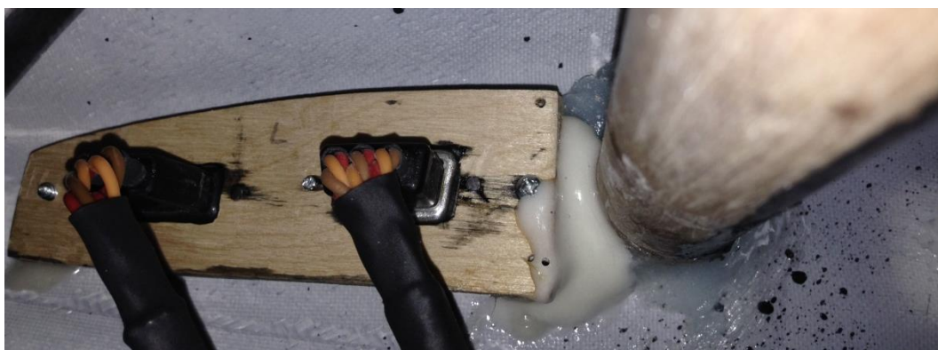
Figure 28. Servo-connector support glued into position with epoxy mixed with fiberglass flock to strengthen the joint.
